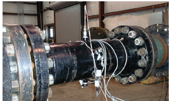
Figure 6. Test spool and thermowells installed in CEESI flow test pipe.
